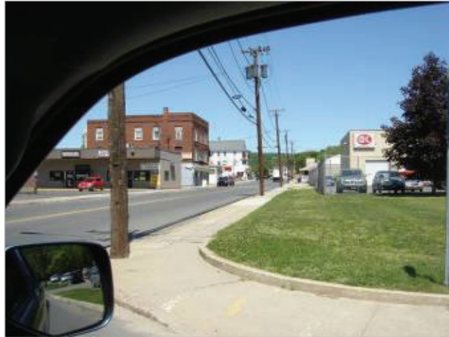
Utility poles along Thomaston Avenue from Boyden Street
