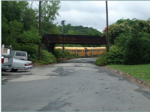
Jackson Street railroad trestle existing conditions
