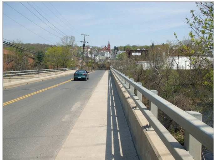
Washington Street bridge looking east
