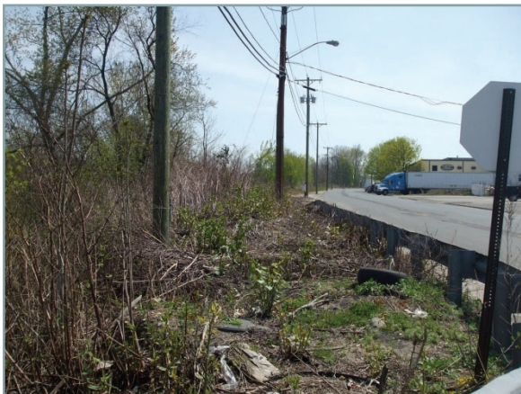
Railroad Hill Avenue existing conditions
