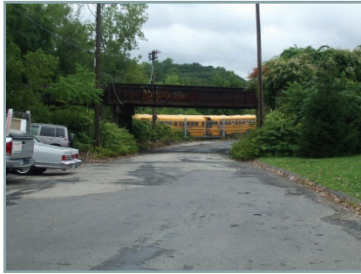
Jackson Street railroad trestle existing conditions
