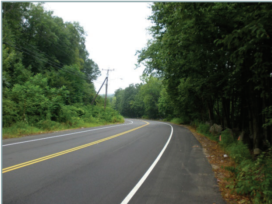
Platts Mills Road existing conditions
