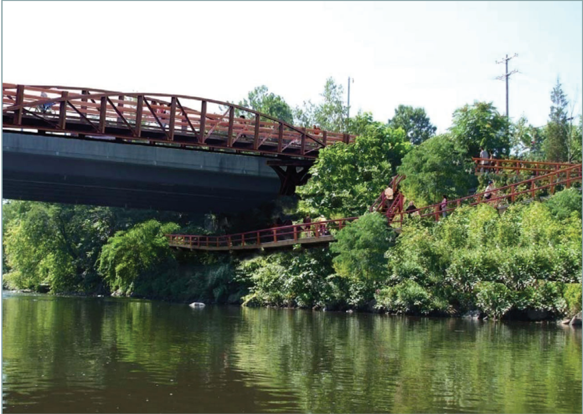
View from the river of the Huntingdon Avenue bridge featuring the new greenway bridge and the greenway passing below it and the existing structure
