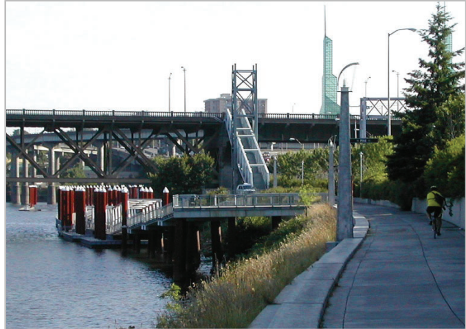
The Eastbank Esplanade in Portland, Oregon illustrates one way for a trail to be cantilevered over water to avoid a significant barrier.
