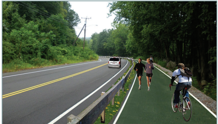
The travel lanes and shoulders along Platts Mills Road could be narrowed to provide space for the greenway trail.
