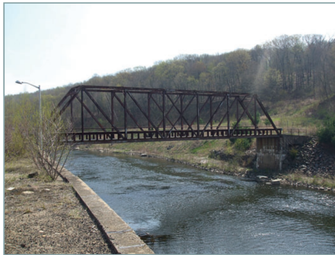
The existing steel truss bridge offers a unique opportunity to access the open space and fishing holes along the west bank of the river. (Grant money for improvements is being sought by the City)
