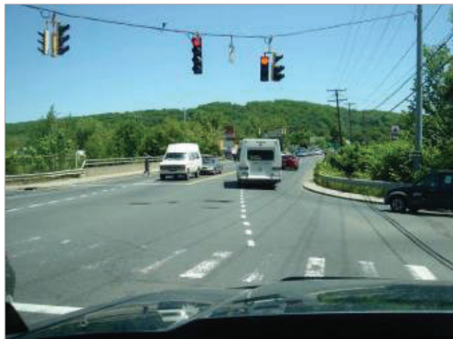
Traffic signal heads at the Huntingdon Avenue bridge
