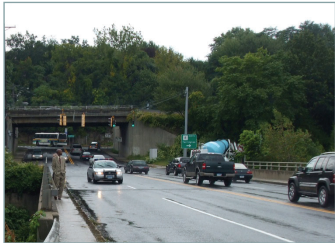
Huntingdon Avenue bridge looking west to Route 8
