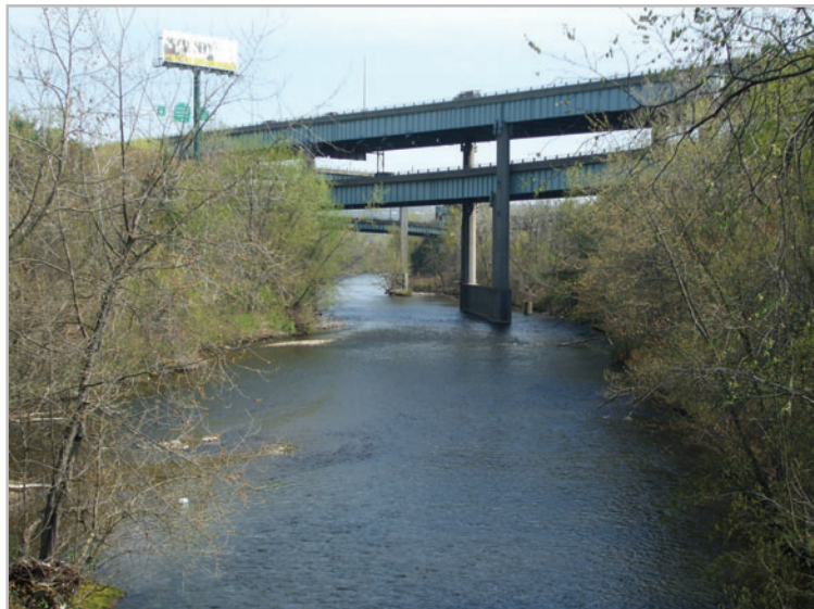
The Naugatuck River's corridor of green and blue winds its way below the I-84/Route 8 interchange.
