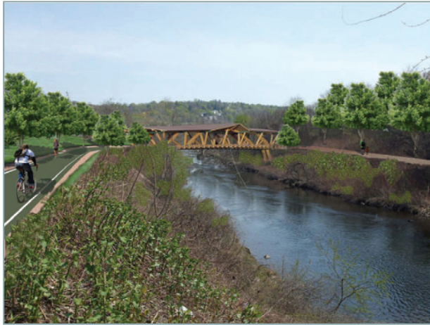
a more innovative covered bridge;
