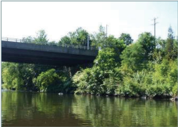
Huntingdon Avenue Bridge existing conditions
