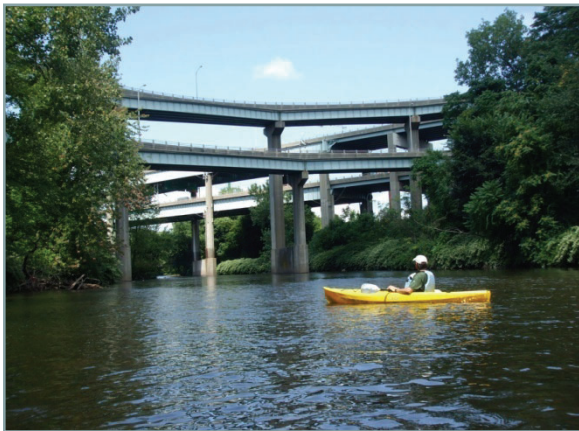
Area south of I-84/Route 8 interchange existing conditions
