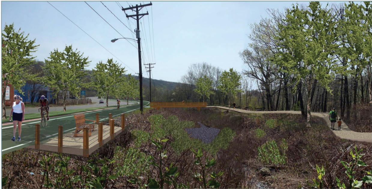
With the removal of a travel lane, a portion of South Main Street could accommodate the greenway trail and a landscaped buffer.
