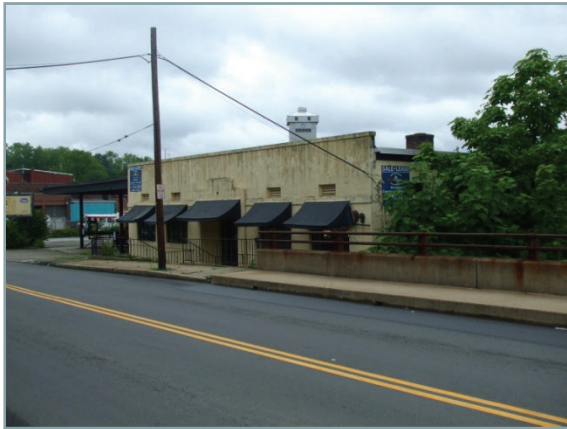
West end of the Eagle Street bridge existing conditions
