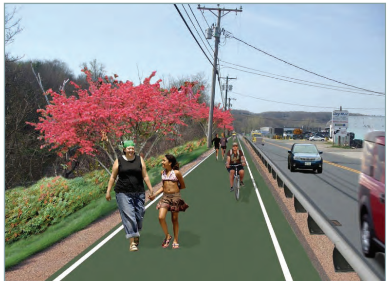
Narrowing the wide travel lanes along Chase River Road provides the necessary space to accommodate the greenway trail and adjacent crash barrier at the top of the river bank.
