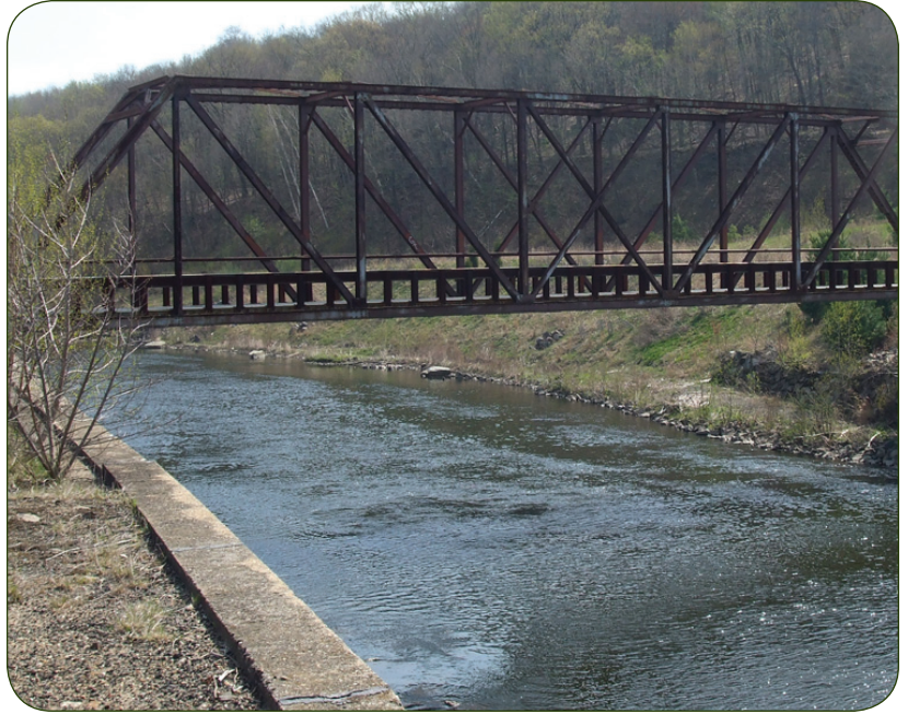
The existing steel truss bridge offers a unique opportunity to access the open space and fishing holes along the west bank of the river.
