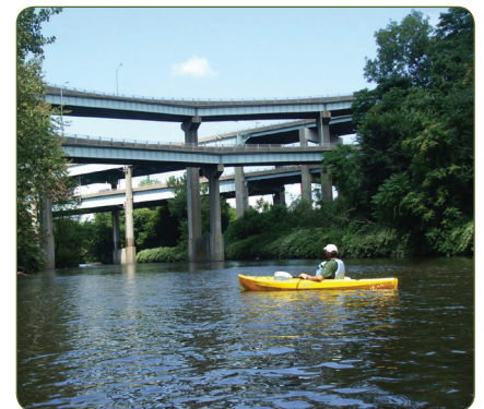
Mixmaster existing conditions
