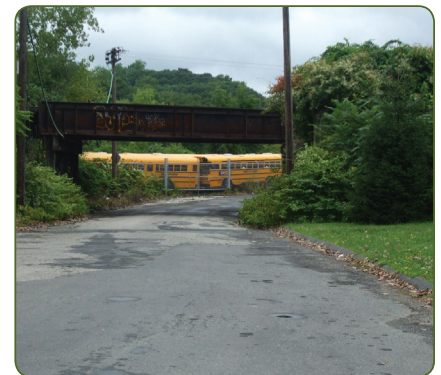
Jackson Street underpass existing conditions
