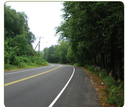
Platts Mills Road existing conditions
